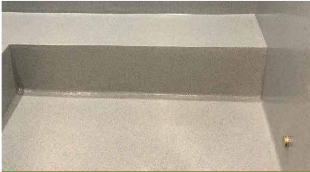
Spa Area with EPO-Guard™ TRQ Troweled Quartz System
